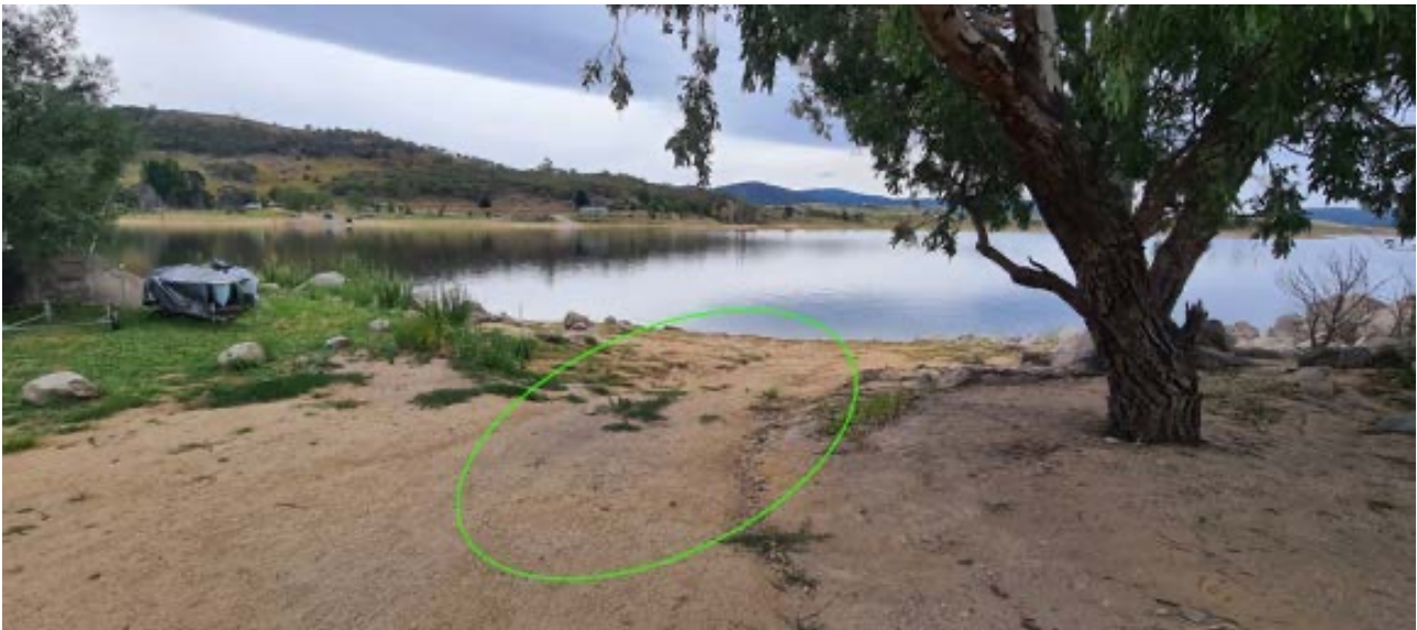
Fig 3. Sailing Club boat ramp is badly eroded and is not used as it is considered unsafe.
